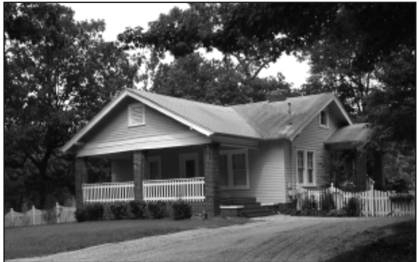
Except for the changed porch rail, the Brewer house looks almost exactly as it did when built in 1923.
