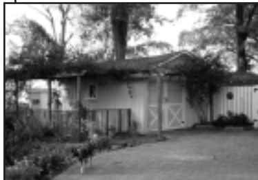
The garage, above, viewed from two sides, has an automatic garage door disguised to look like its original swinging doors.
